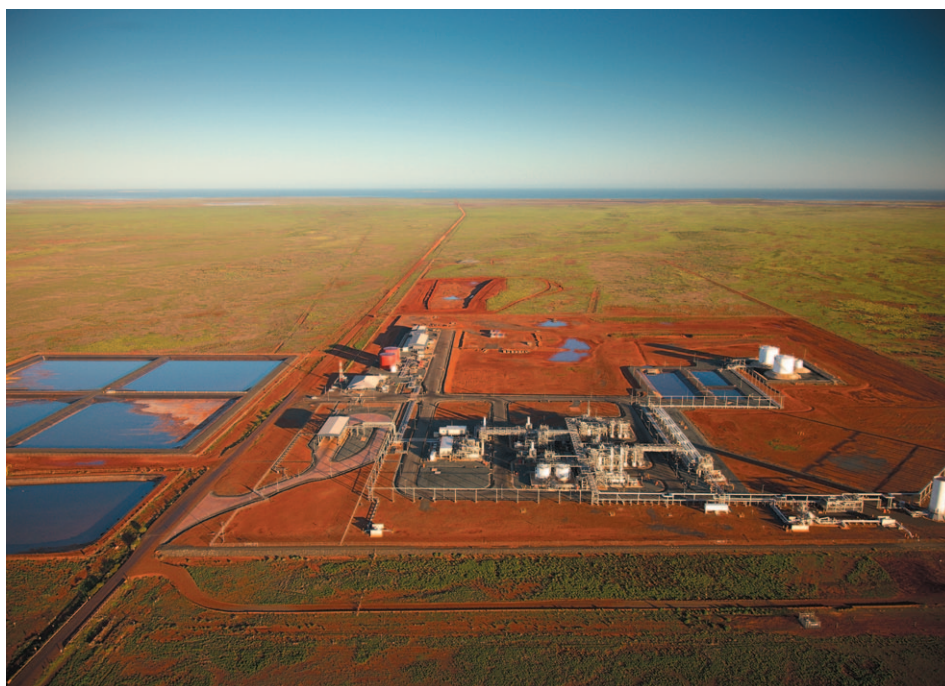
Devil Creek Domestic Gas Plant
