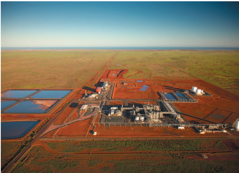
Devil Creek Domestic Gas Plant
