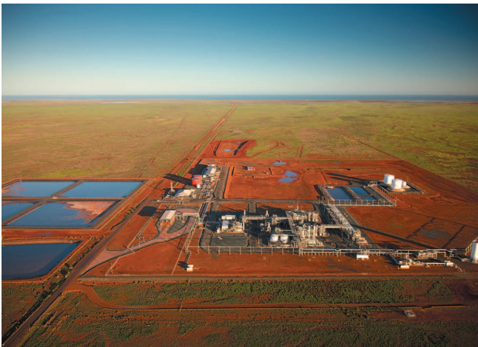
Devil Creek Domestic Gas Plant
